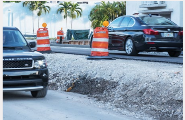
Raised road during construction ( http://www.mbrisingabove.com/ )
