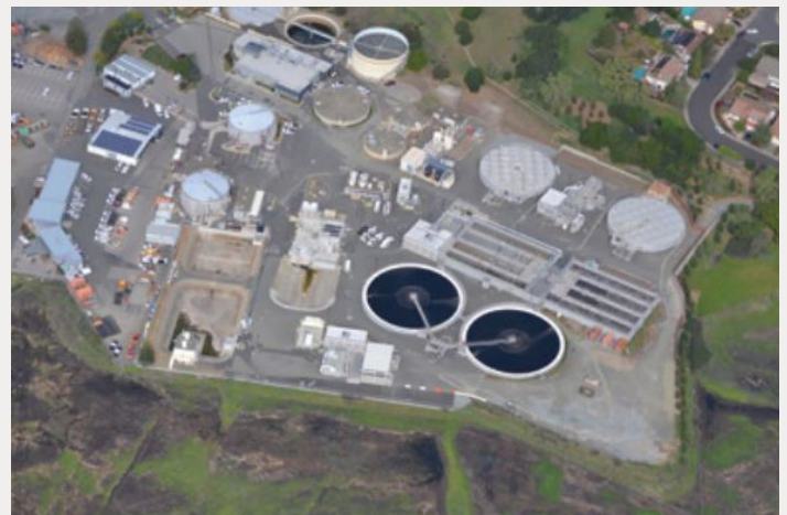
Aerial view of upgraded plant (Novato Sanitary District)
