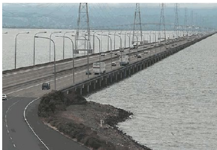
State Route 92 bridge approach heading toward San Mateo (CA COT, 2019)
