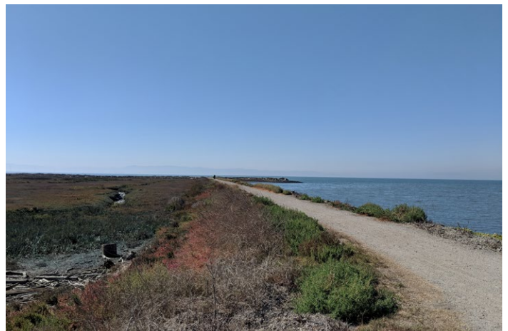
Cogswell Marsh levee adjacent to the Bay (SCAPE Site Photos, 2019)
