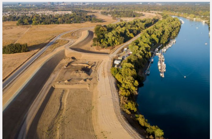
Sacramento River levee
