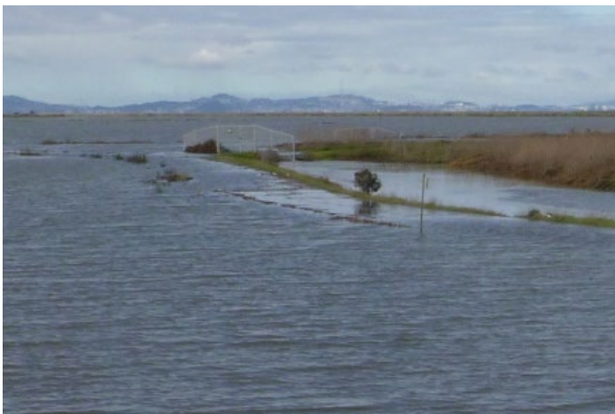
Bay Trail flooding during Jan 2017 King Tide (H.A.R.D., 2017)
