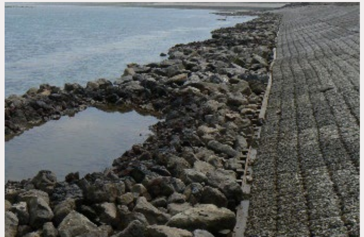
Tidal pool along stabilized revetment ( www.publicwiki.deltares.nl )
