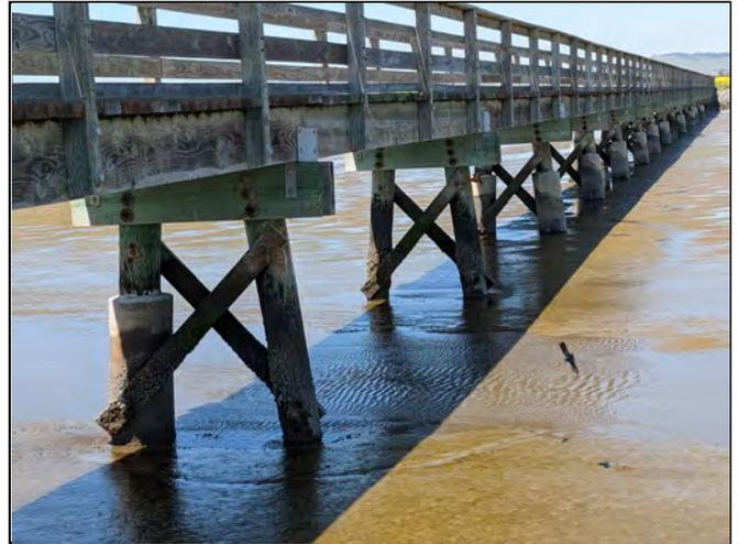
Description: Repair damaged bridge timber piles with fiberglass jacketing and epoxy mortar. Repairing the two bridges will take place over several years to work within the tidal and environmental constraints.
