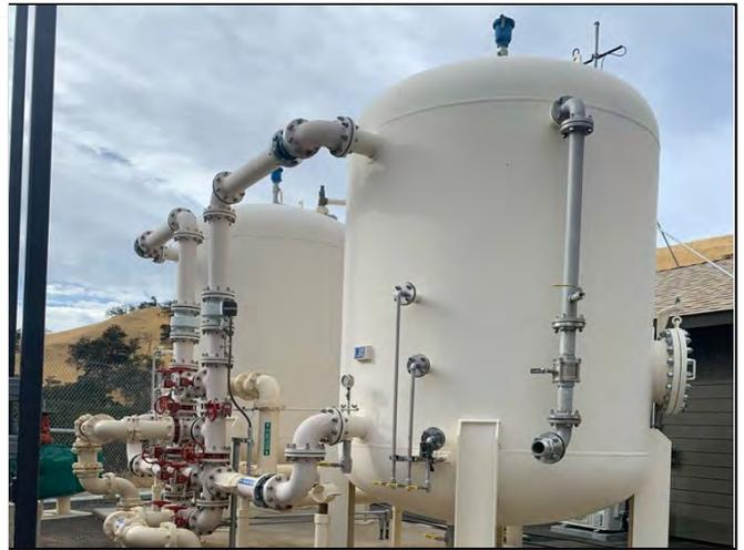
Description: Stabilizing the water system includes, repair the solids contact clarifier, replace several six inch control valves in the main water distribution system, repair the raw water intakes, remove silt, and major filter repack and renovation.
