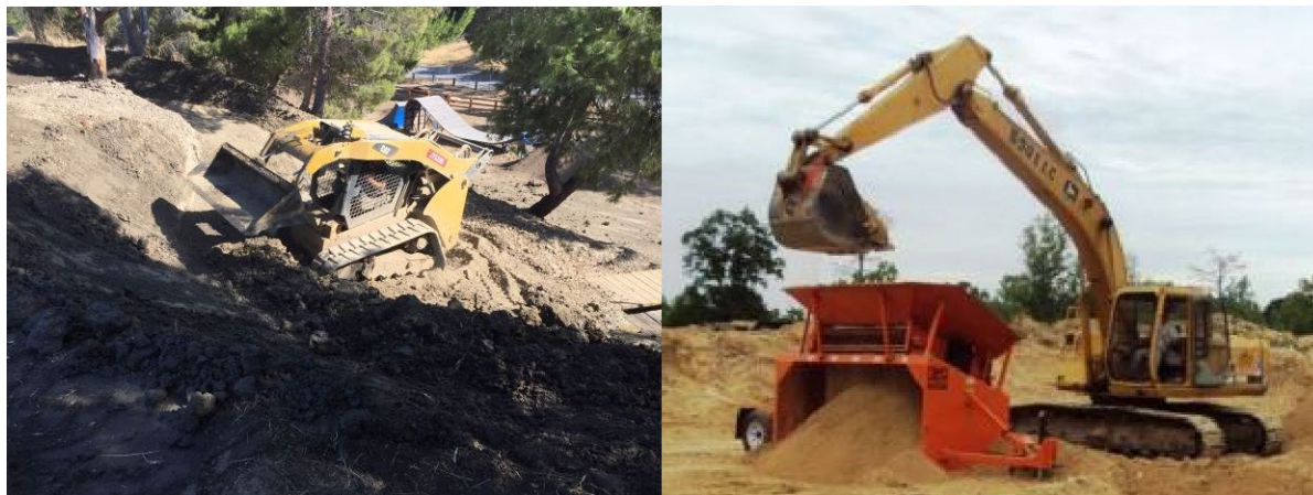
Conditioning a larger work area with a skid steer. Conditioning a soil stockpile with an auto sifter.
