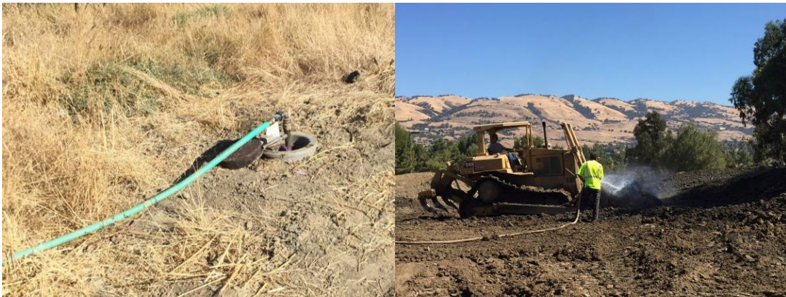
Using the quick couple network onsite moisture condition soil prior to beginning work.
