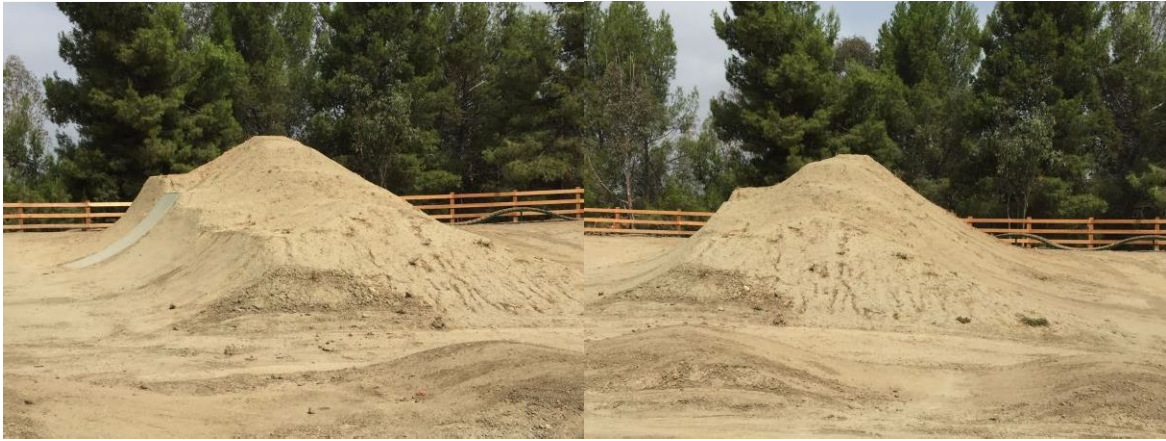
Final shape jump set with kicker lip on the front end and a lander transition on the back end.
