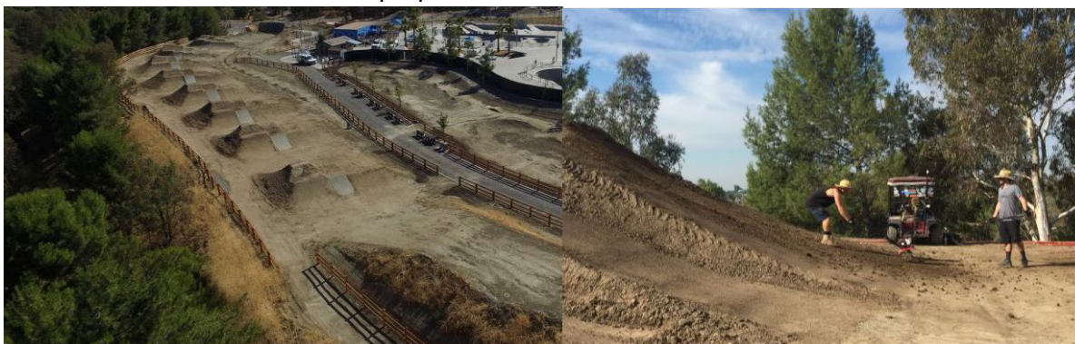
Finished jump set. Using a tiller to condition soil and fine tune landing.
