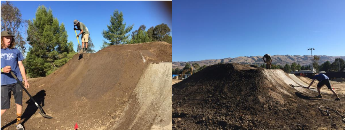
Using shovels to pack and shape dirt jump lip. Using the concrete kicker to shape to.
