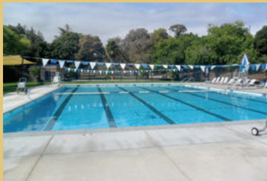
Ambrose Park refurbishment, Bay Point $1,127,177
