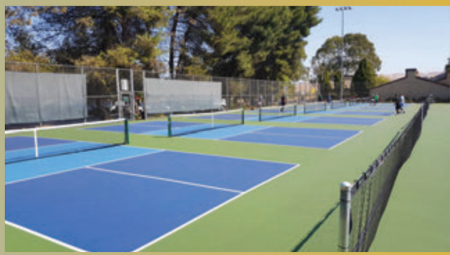
Tennis Courts resurfacing, Concord $90,916
