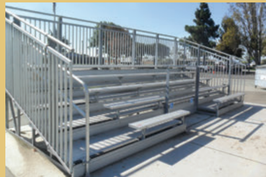
Stenzel Park bleacher replacement, San Leandro $96,000
