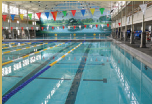
Richmond Plunge Natatorium renovation $3 million
