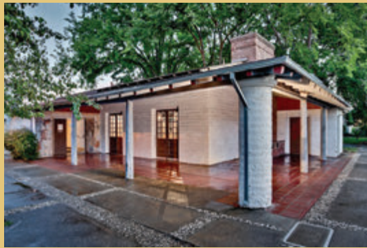
HARD Adobe Art Center, lighting and security upgrades, Castro Valley, $25,860
