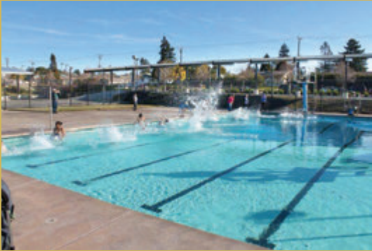
HARD Castro Valley Swim Center renovation $1.5 million
