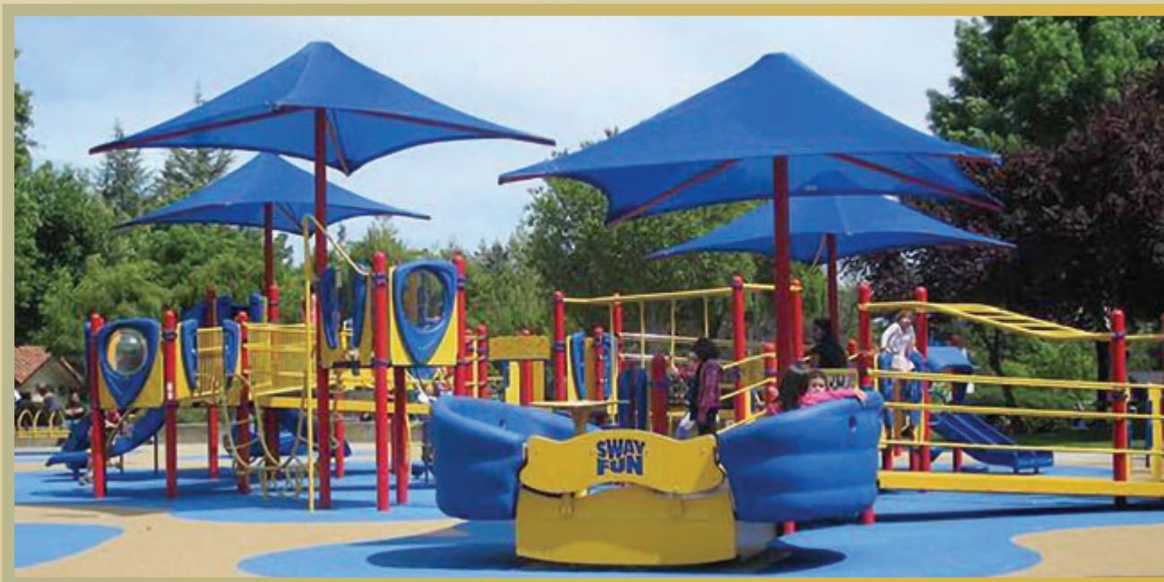
Athan Downs Playground renovation, San Ramon $305,701
